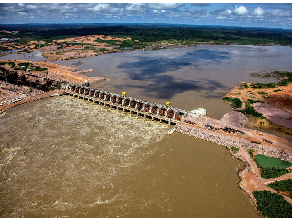
The Jirau Dam on Brazil's Madeira River has enormous impacts, as will planned dams, in displacing human populations; blocking fish migrations; and provoking biodiversity loss, greenhouse-gas emissions, and so on.
